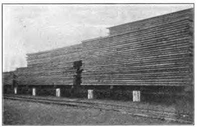
Fig. 83.—Another type of permanent foundation. Steel rails are embedded in concrete piers. The lumber is fully  $2\frac{1}{2}$  feet above the ground, insuring excellent ventilation.
